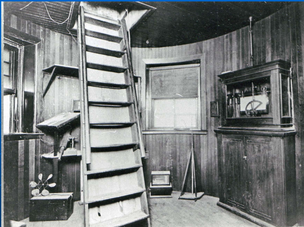
Second floor of old tower after sheathing
