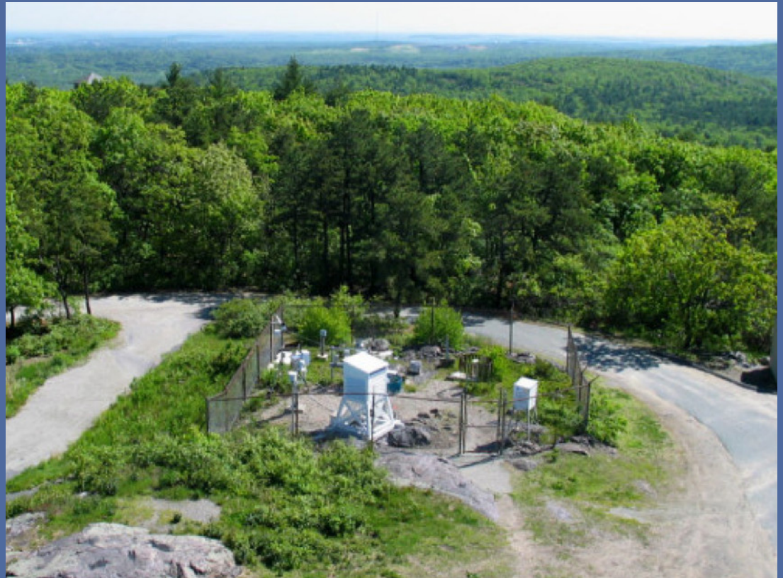
Outdoor instrument enclosure at BHO
